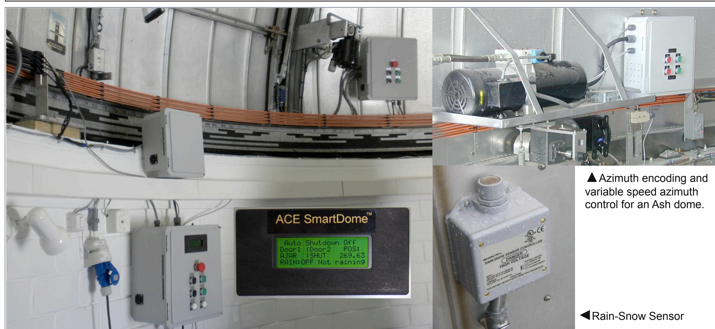
▲ The observatory enclosure is managed with an ACE SmartDome™ which is a fault-tolerant system to handle two shutter doors and up to 6 other devices, such as windscreens, platforms and observing cages. It integrates with rain-snow and cloud sensors to provide autonomous shutdown. It will also close a dome if communication is lost. The azimuth is equipped with either absolute or incremental encoding and has ramp-up/down speed control. The system has been deployed on roll-off roofs and classical domes up to 25m diameter.
